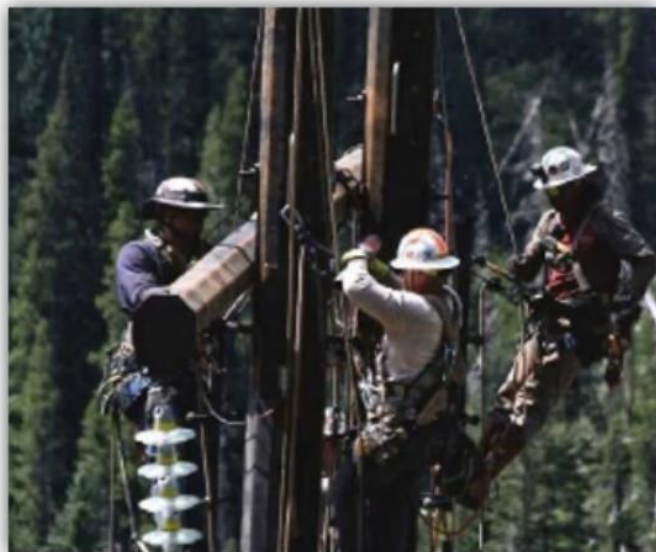
Linemen being lowered into a transmission pole
