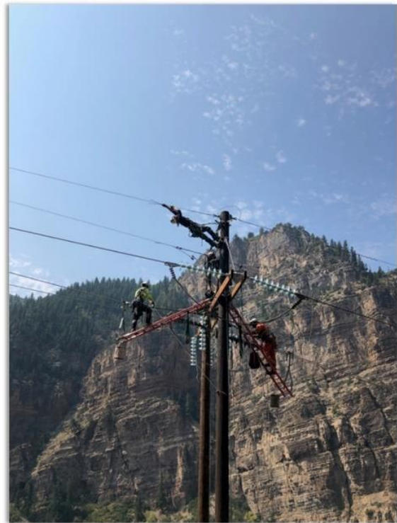
Linemen working on transmission line
