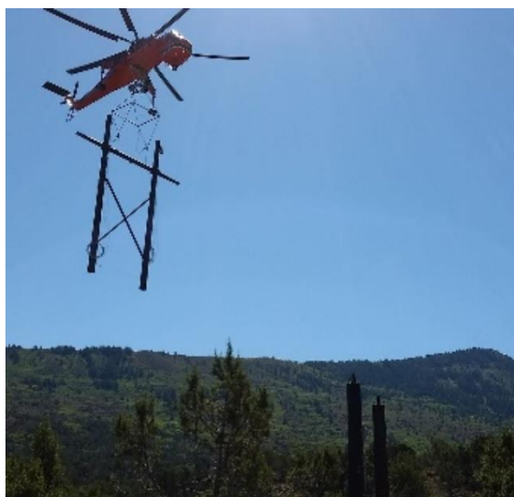
Helicopter flying in replacement poles
