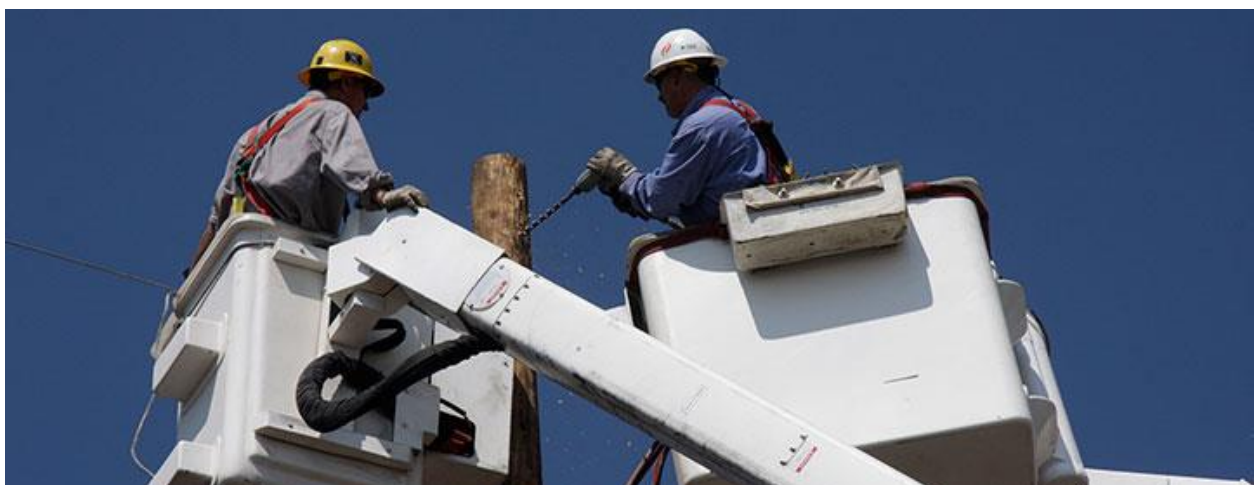
Linemen repairing a distribution pole
