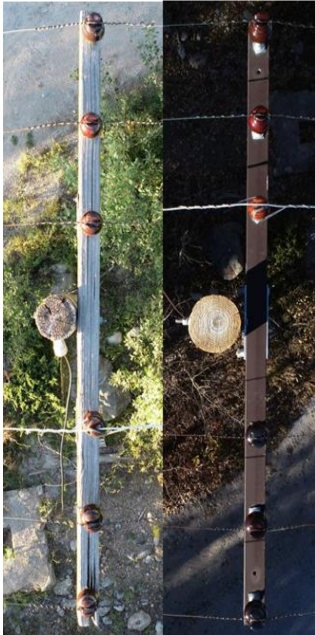
Pole top repair (before and after)
